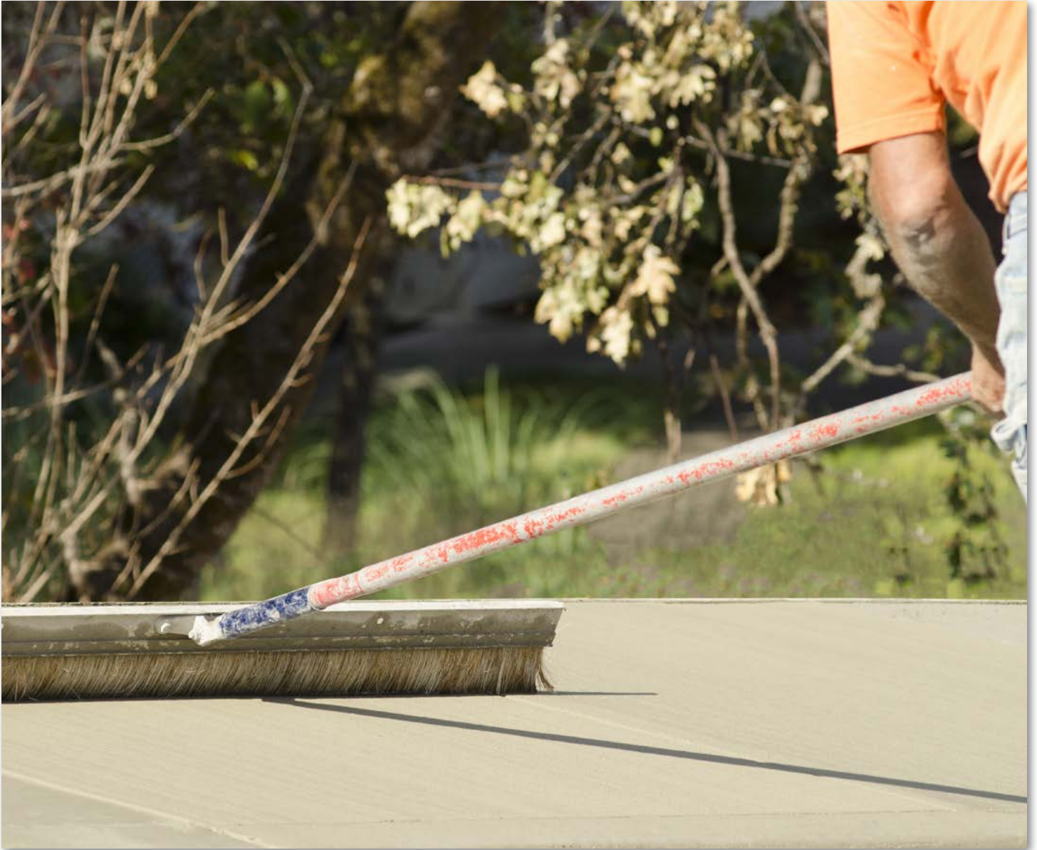
Contractor broom finishing a concrete sidewalk/curb
