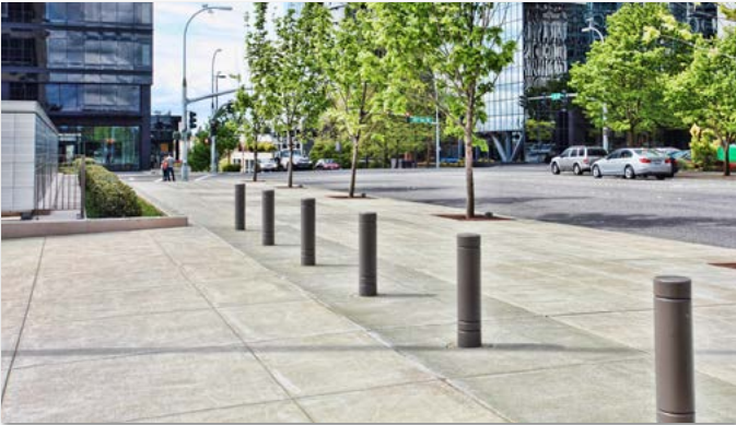
High Traffic Walkways
